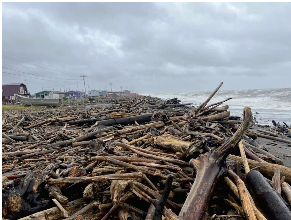
Figure 10. Shaktoolik's berm destroyed in the storm
